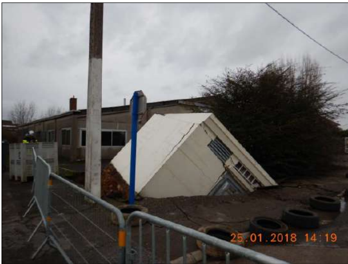
Figure III.21: Effondrement route de Tilloy. Source: DDTM62
